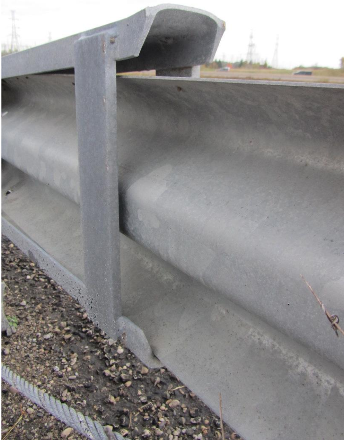
Figure 11: View of the ET-PLUS terminal on October 14, 2014. Note that the substantial difference in the horizontal angle of the terminal and guardrail causes the bottom edge of the rail to rest on the bottom of the channel while there is a large gap at the top.
