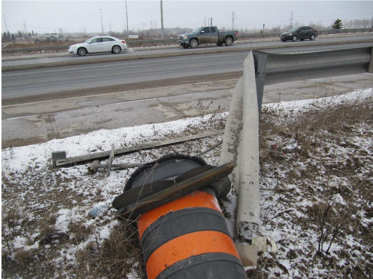
Figure 22: View showing that the end of the guardrail has been bent at its anchorage post however there is little evidence of additional damage to it.
