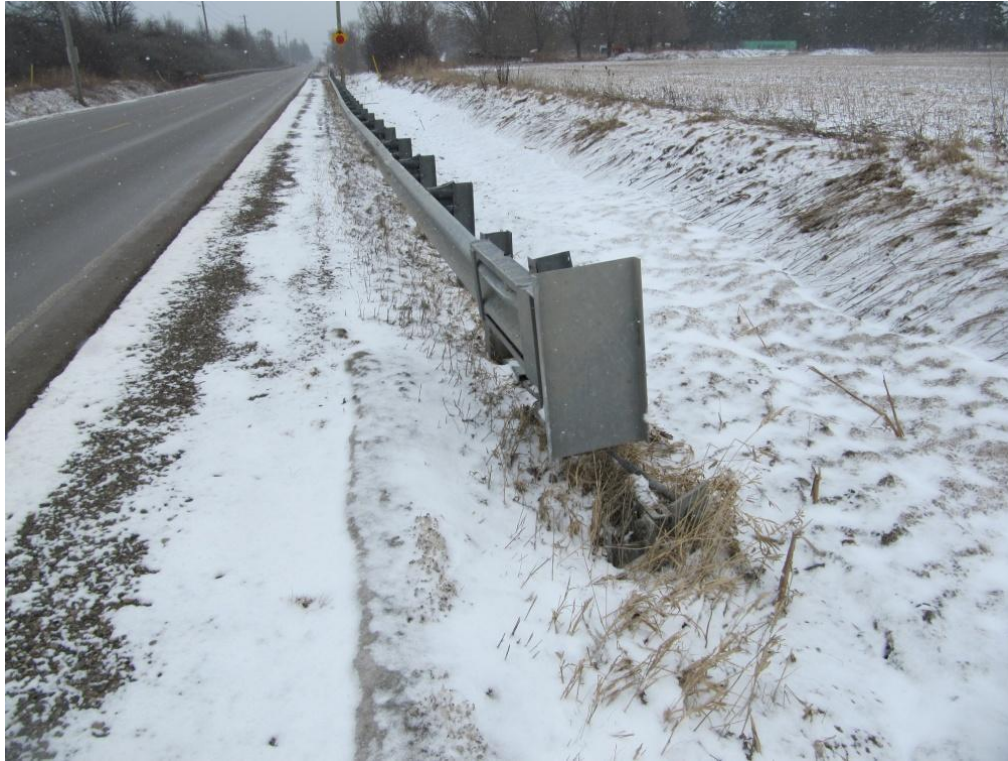
Figure 28: View of the ET-PLUS terminal and guardrail initially suggests there is no damage to it.
