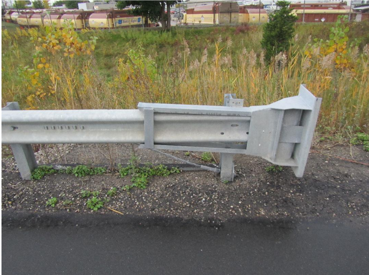
Figure 2: Side view the ET-PLUS guardrail terminal showing the plate (head) on the right and the channel attached behind it. The end of the guardrail fits within the channel.
