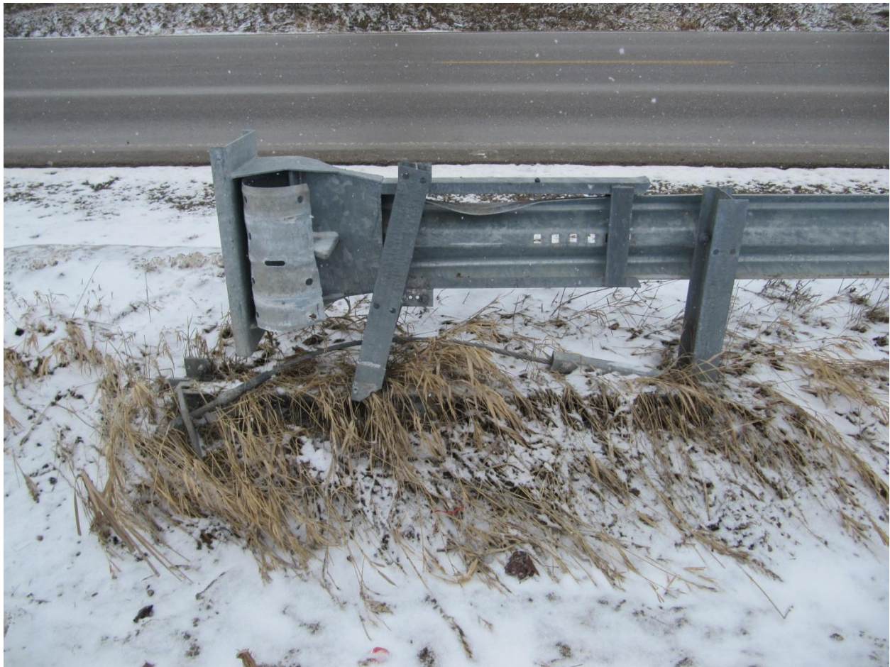
Figure 30: A ditch-side view of the terminal indicates that a small length of the guardrail has passed through the terminal head and has been extruded out of its side.
