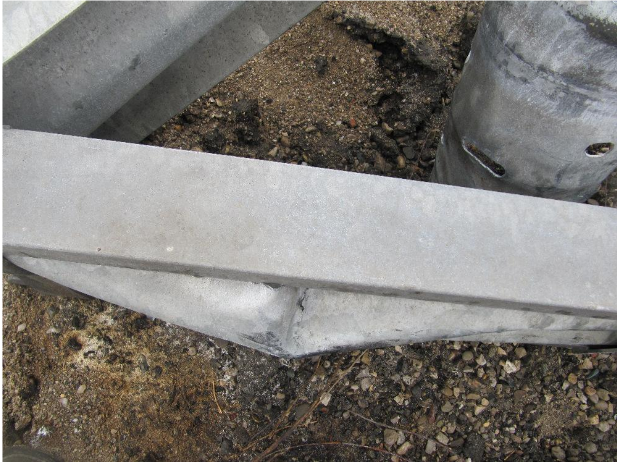
Figure 18: View looking down at the guardrail within the channel showing how it is deformed and is protruding out of the side of the channel.
