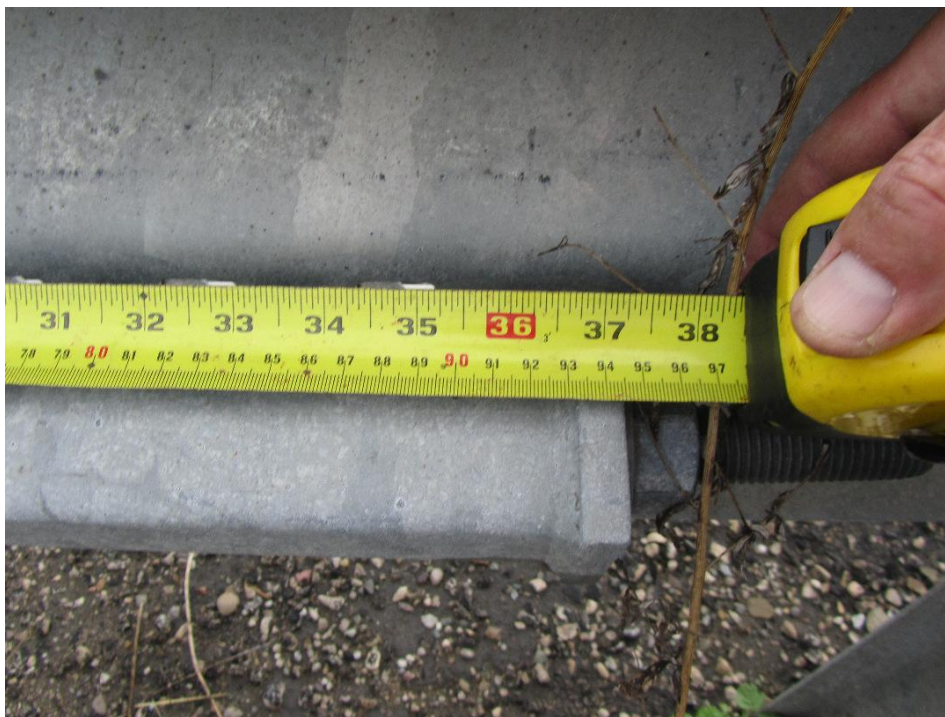
Figure 13: View showing that the measured distance to the rear edge of the anchor bracket is about 37 inches.
