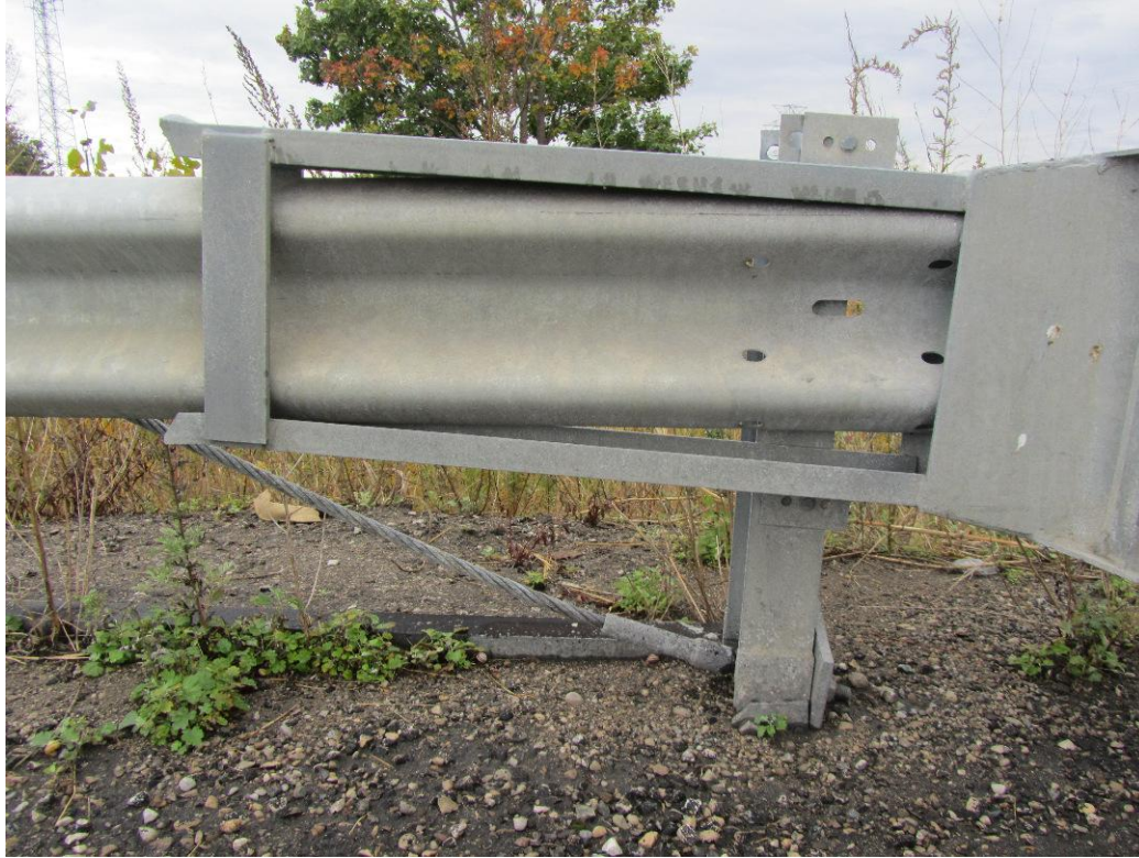
Figure 8: Note the substantial difference in the horizontal angle of the head and channel of the ET-PLUS versus the angle of the guardrail.
