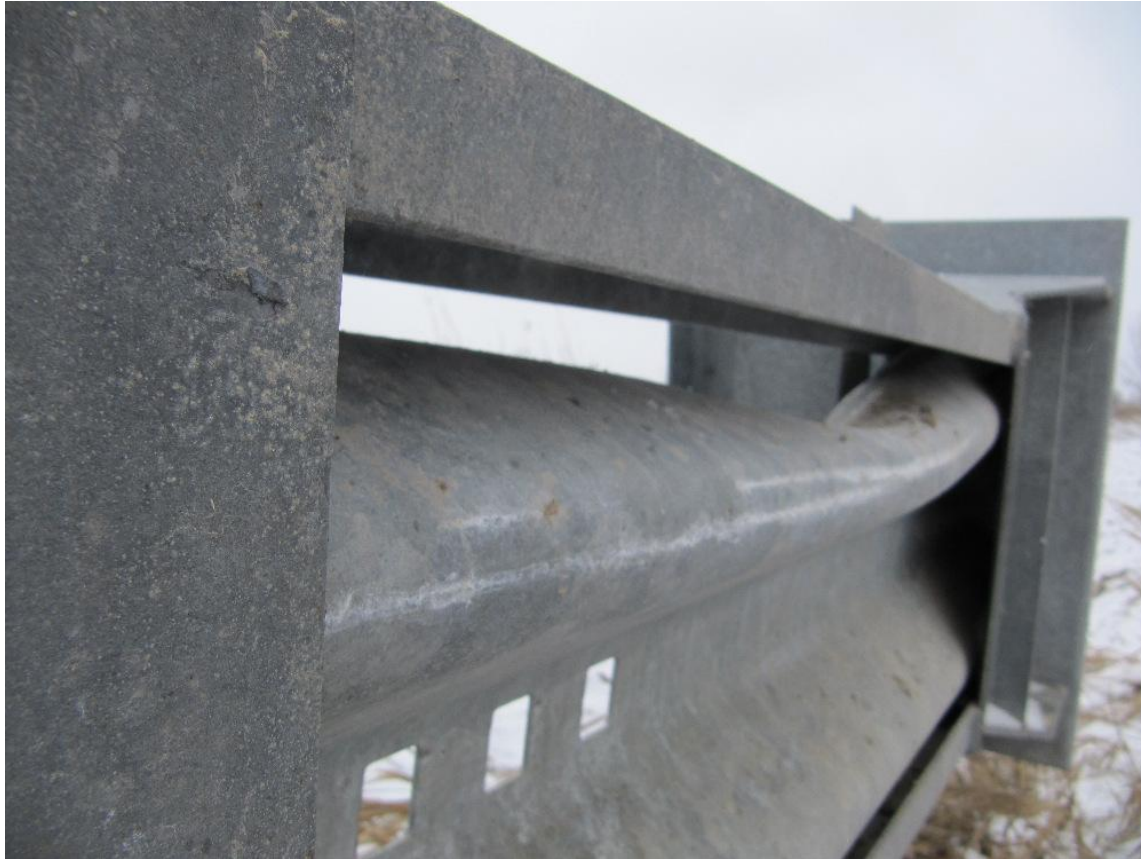
Figure 32: View of a light-coloured scrape on the rail that extends from the rear vertical bar of the channel through to the terminal head.
