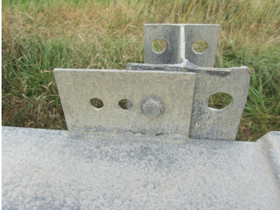
Figure 36: Opposite view showing the anchorage bracket extending from the terminal and how a single bolt attaches the bracket to the vertical anchorage post.
