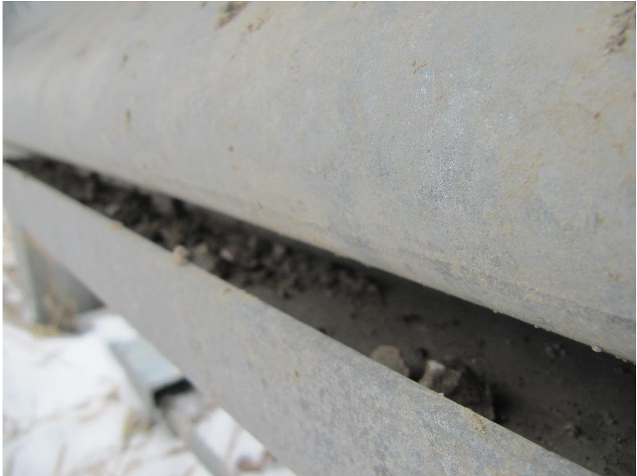
Figure 33: View of gravel resting along the bottom of the terminal channel. Such debris could help in restricting the sliding of the channel and head along the rail or it could become jammed in the narrow opening of the terminal head.
