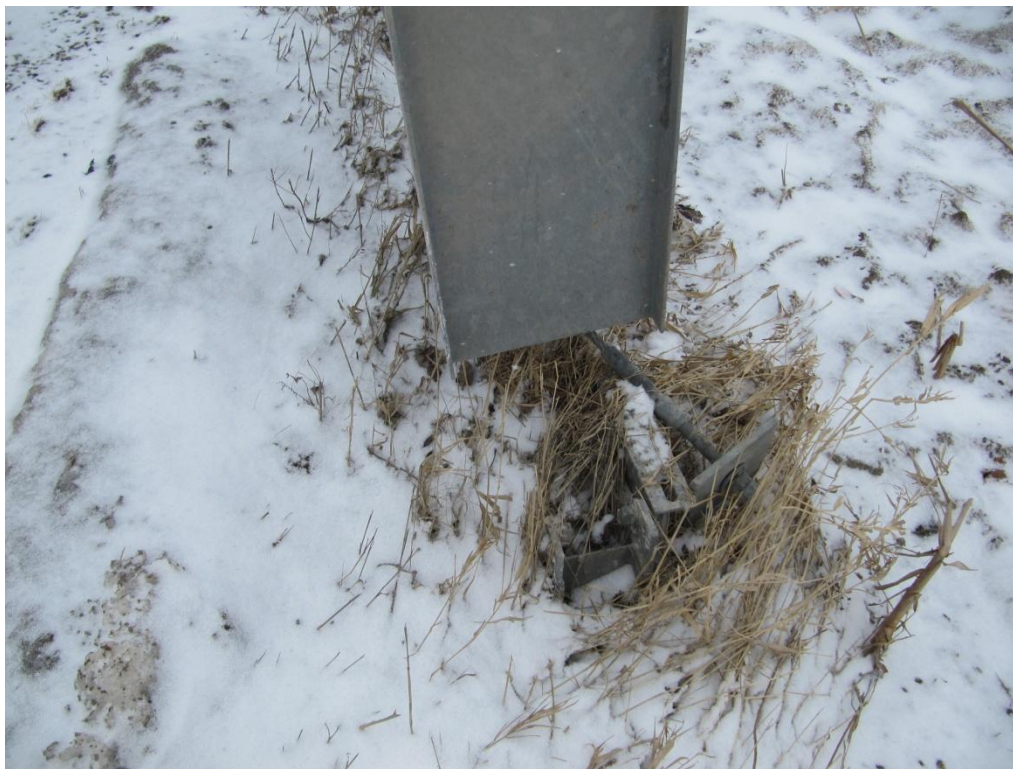
Figure 29: View of the anchorage bar that normally lies beneath and behind the terminal head. Since the head is behind the forward end of the bar it clearly indicates that the terminal has been pushed backwards.
