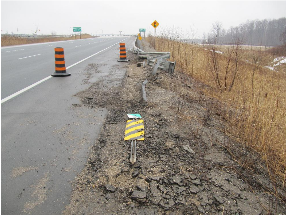
Figure 7: Overall view of damaged ET-PLUS terminal including a substantial length of guardrail.
