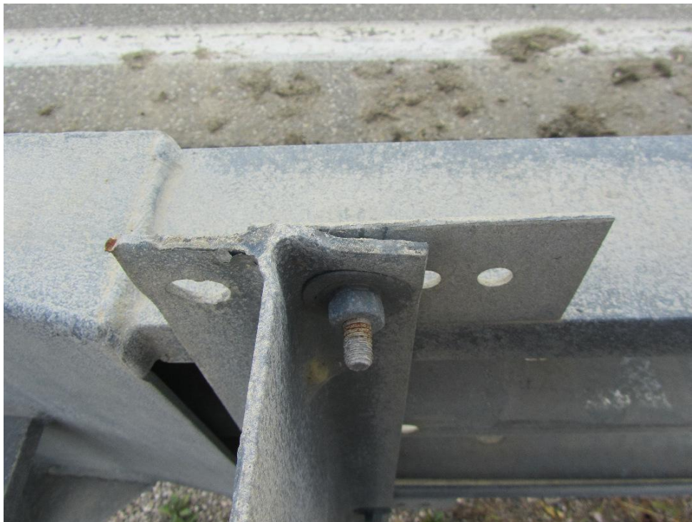
Figure 35: Close-up view of the point of attachment of the terminal to its vertical anchorage post.
