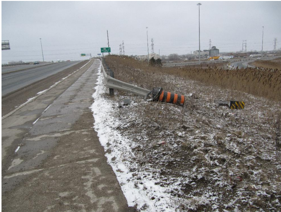
Figure 21: Closer view of the damaged guardrail end.
