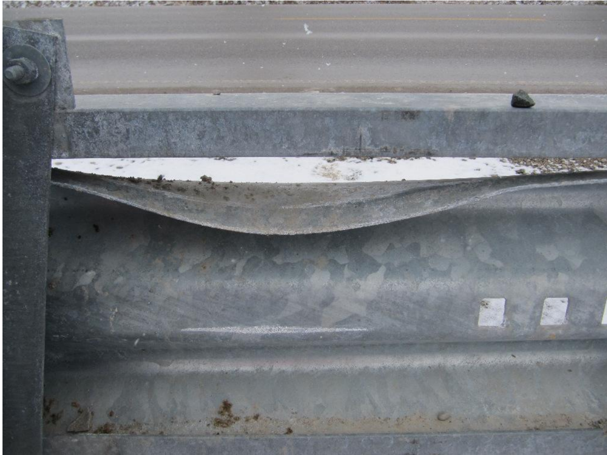
Figure 31: View of an unusual deformation to the top of the guardrail in the vicinity where it is encompassed by the channel of the terminal.
