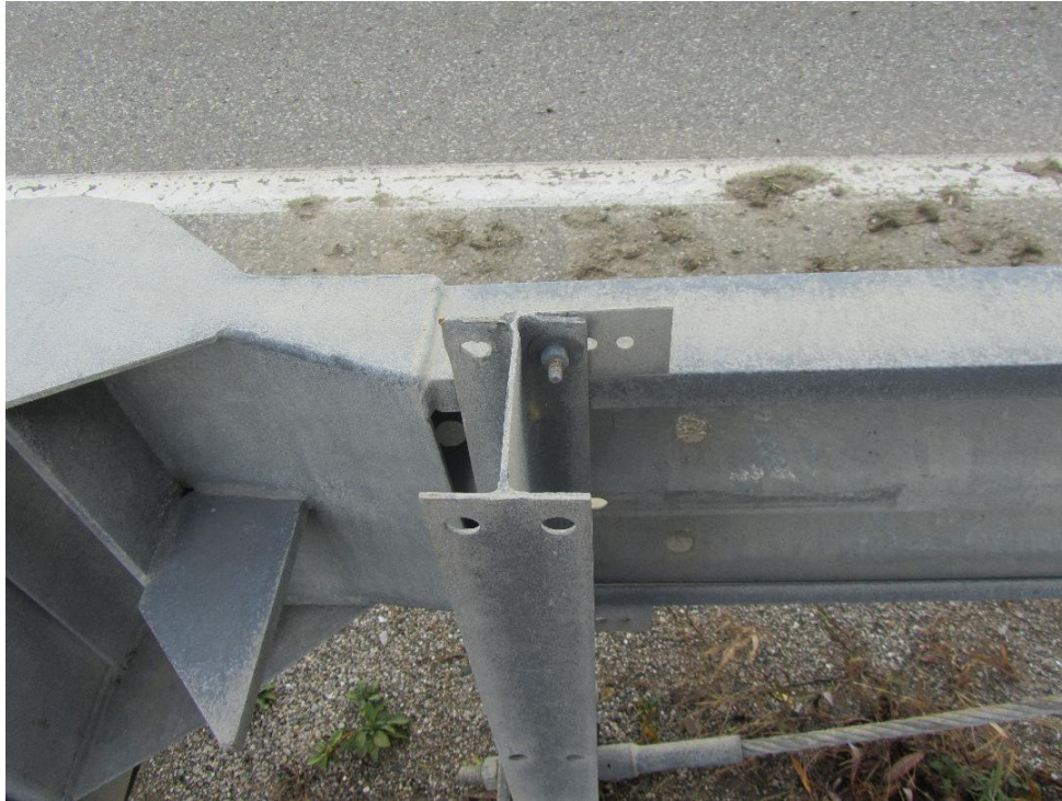
Figure 34: View of an ET-PLUS installation on Ilderton Road near Adelaide Street, north of London, Ontario. This view shows the upper anchorage of the terminal to the vertical anchorage post. A single bolt is the only attachment of the terminal to the post.
